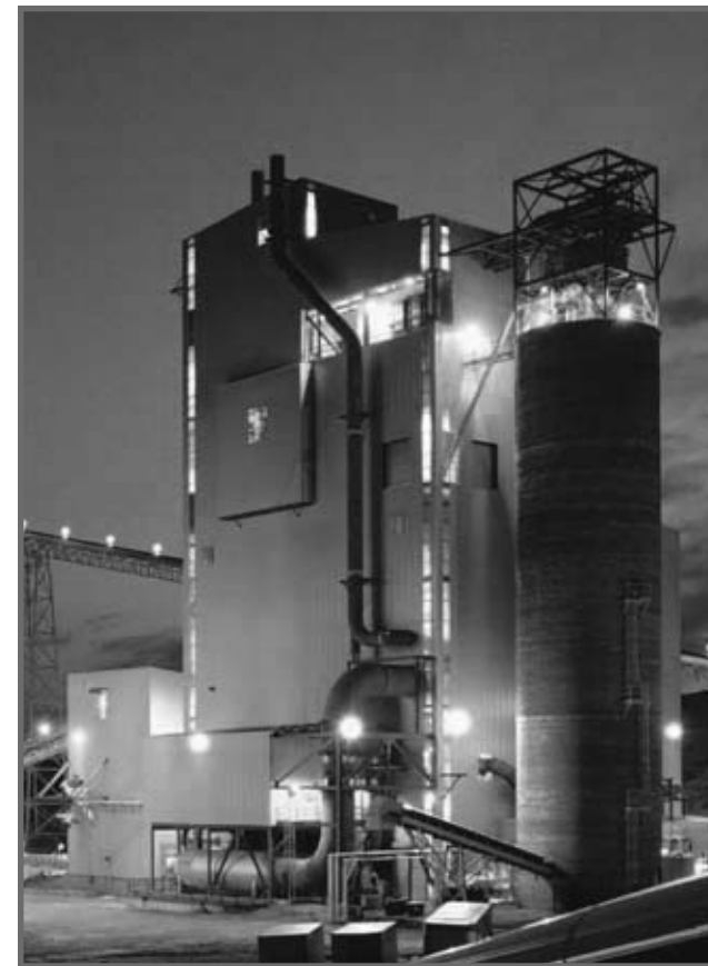
ENCOAL Demonstration Project 1,000 tons per day U.S. Department of Energy/SGI/SMC, Gillette, Wyoming 1992 - 1997 FIG-10
